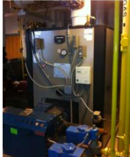
The result is energy savings while ensuring maximum capacity during heavy load periods; this is accomplished with no impact on building comfort levels. Viewed from a perspective of waste heat, the M2G minimizes the waste heat going up the boiler flue while preserving the transfer of beneficial heat into the building.
